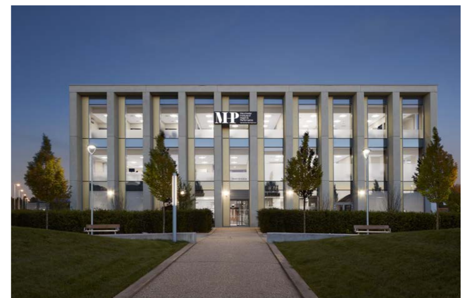
Manchester Institute of Health & Performance - AHR Architects
