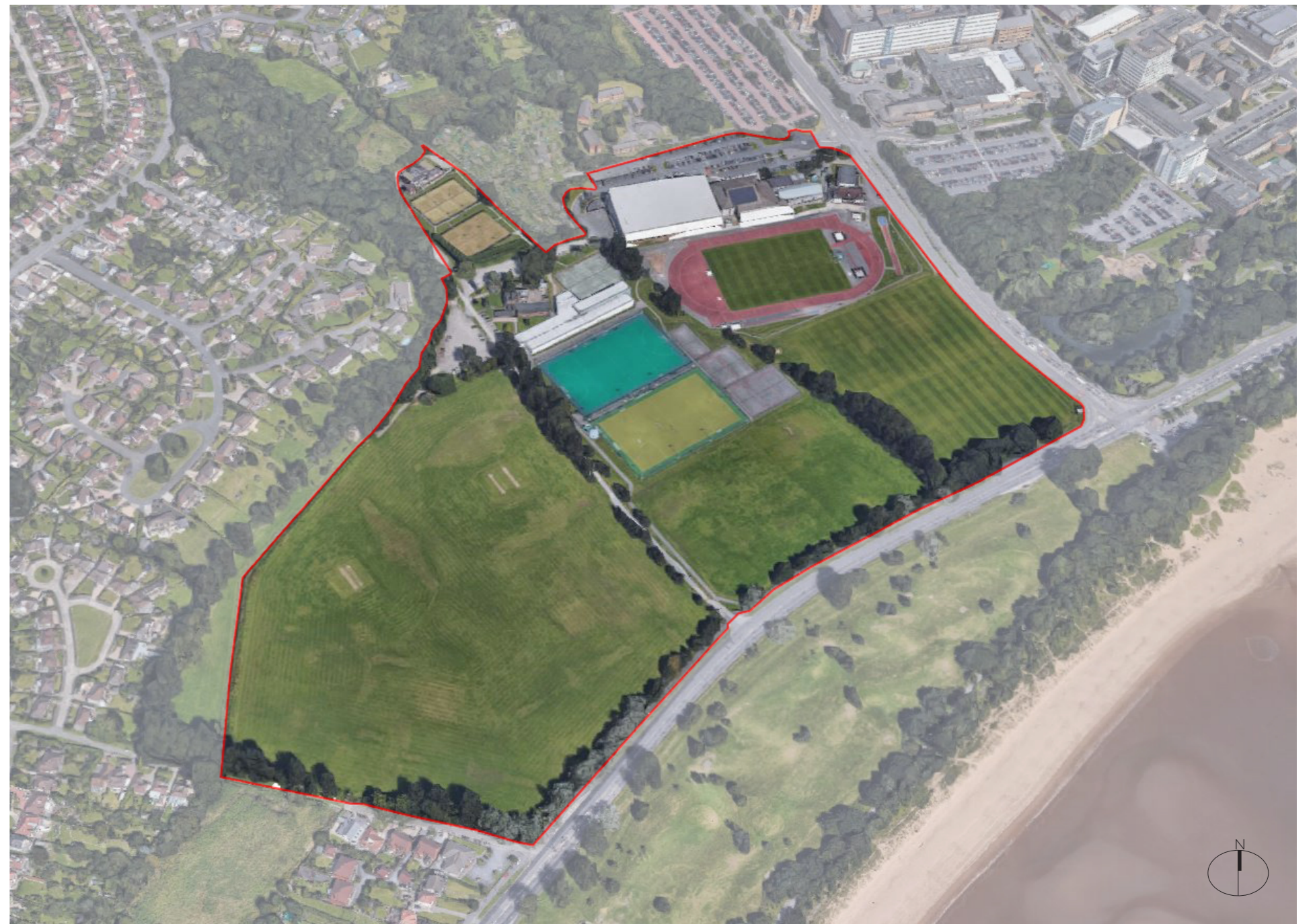
AERIAL VIEW OF SKETTY LANE CAMPUS SITE WITH HIGHLIGHTED STUDY AREA
